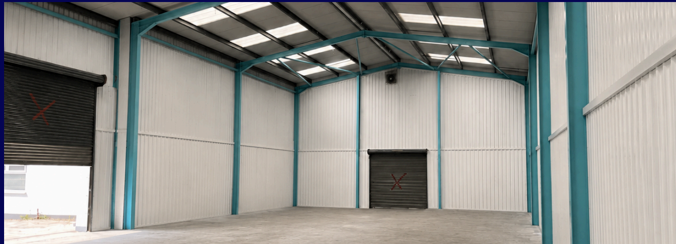
Refurbished warehouse interior
