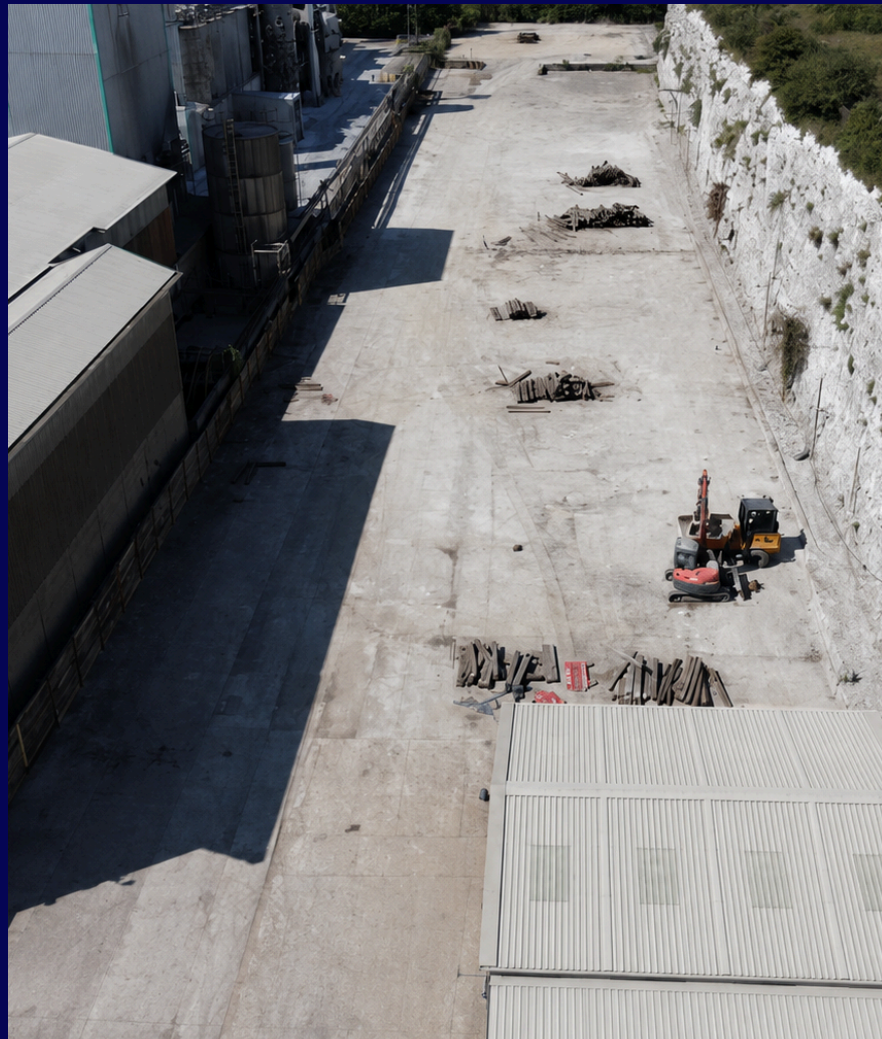
Yard clearance in progress
